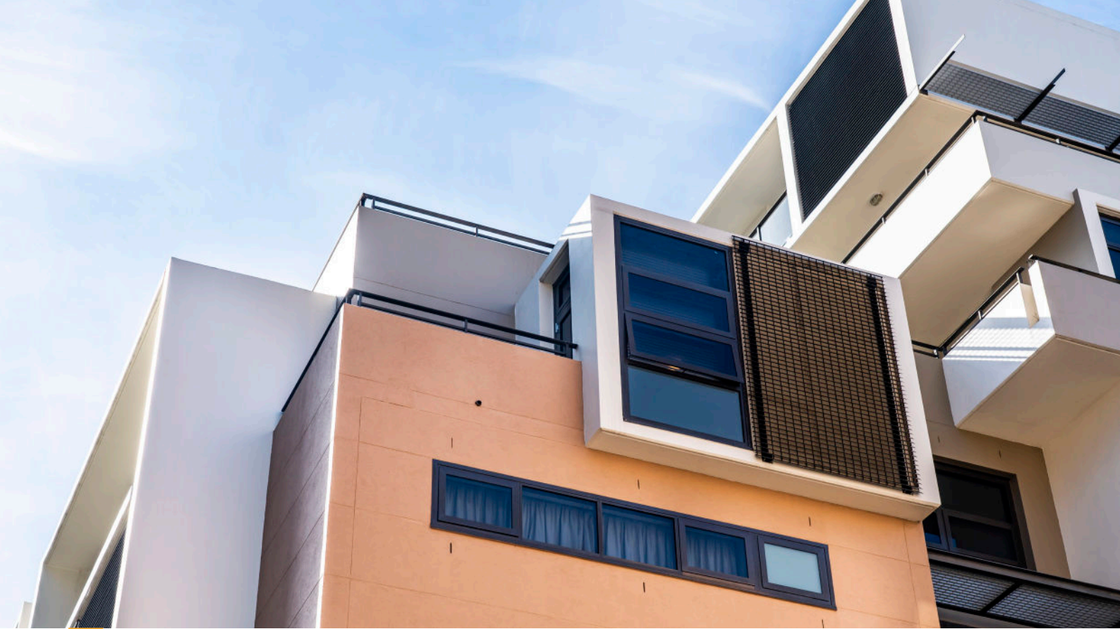
Completed project – Showing our technicians quality workmanship
