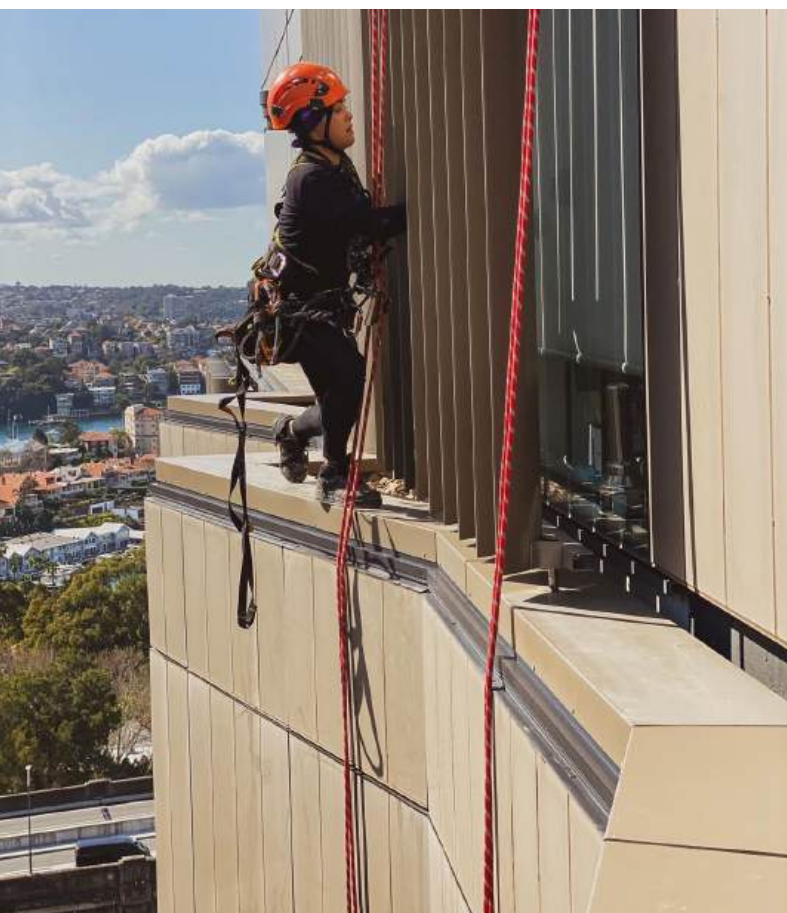
Rope access technicians installing cladding.
