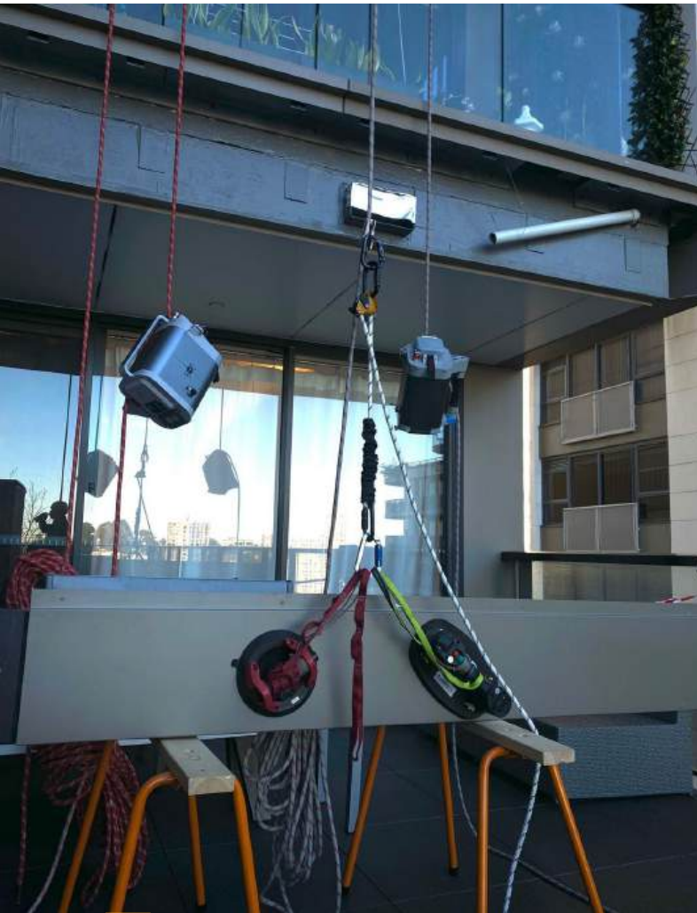
Facade cladding technical rigging for safe transfer from ground
