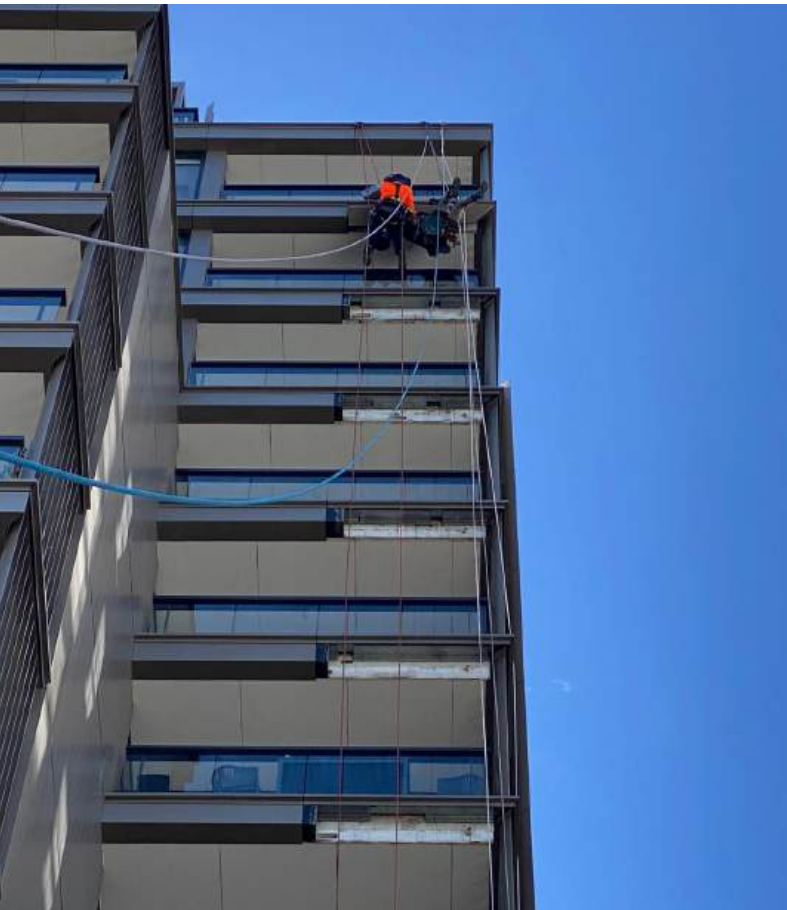
Rope access technicians installing ventilation grills
