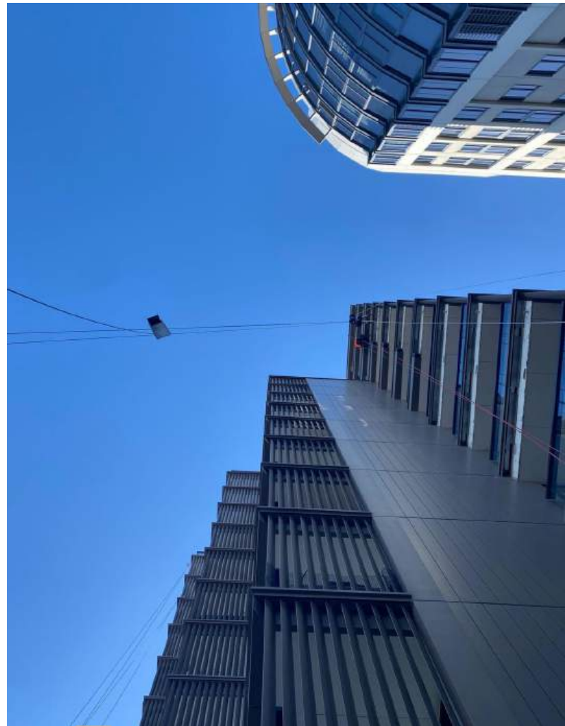
Facade cladding transfer from ground to technicians on the ropes.
