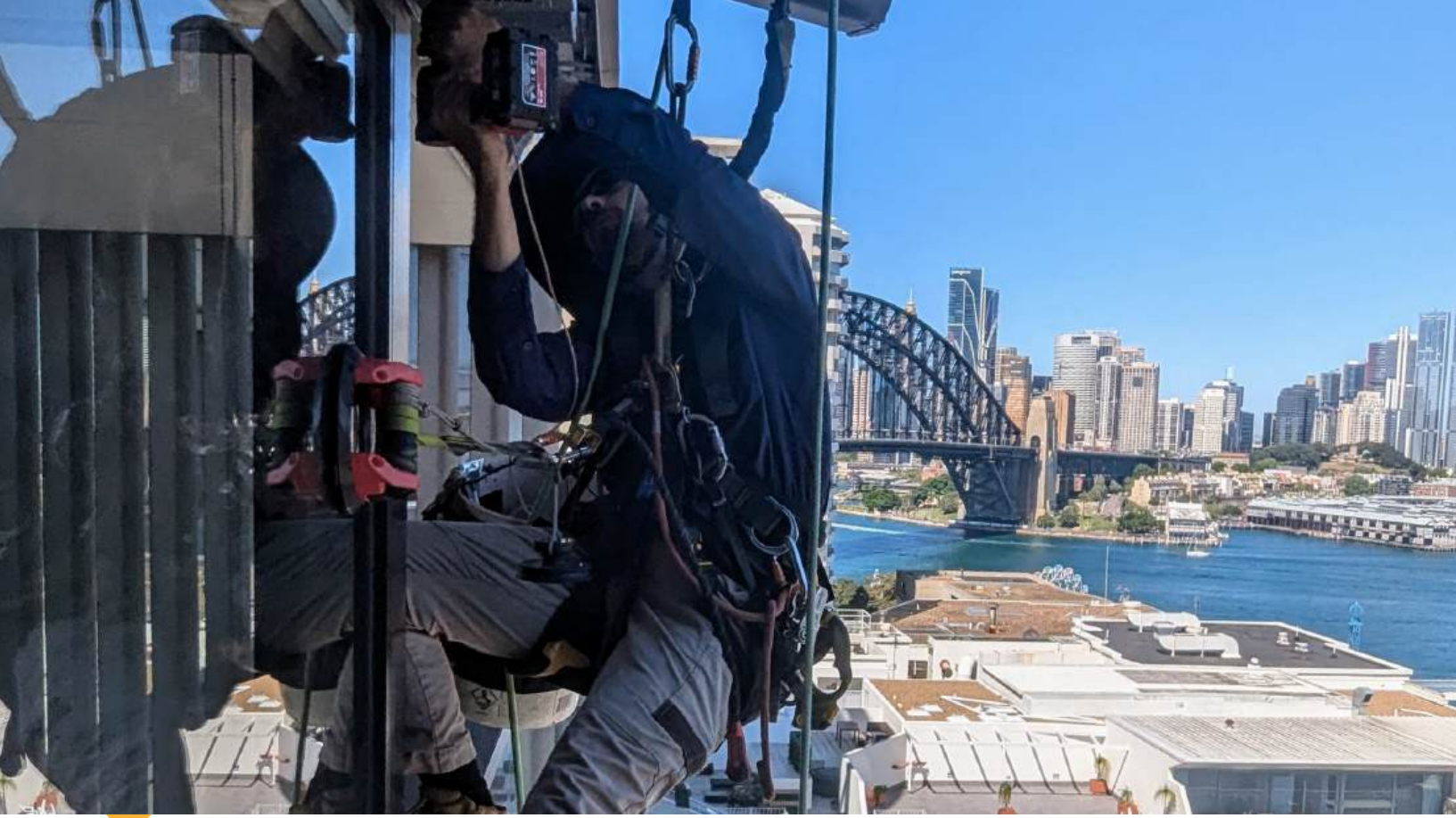
Rope access technicians adjusting gaps in the cladding panel tracks
