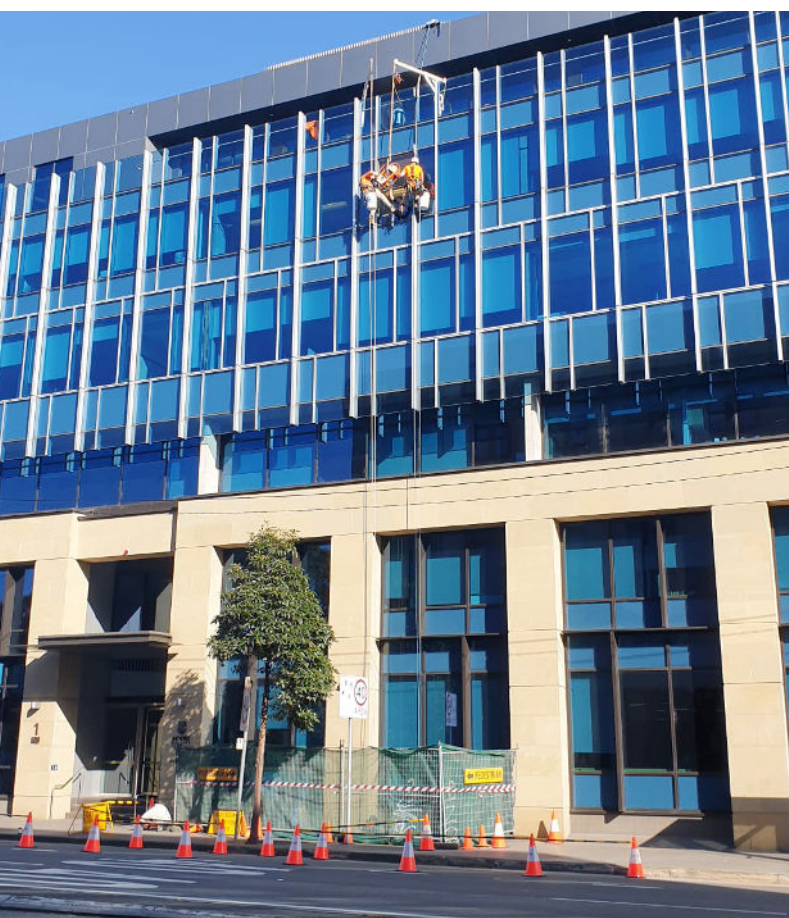
Our Rope Access team removing and installing the glass
