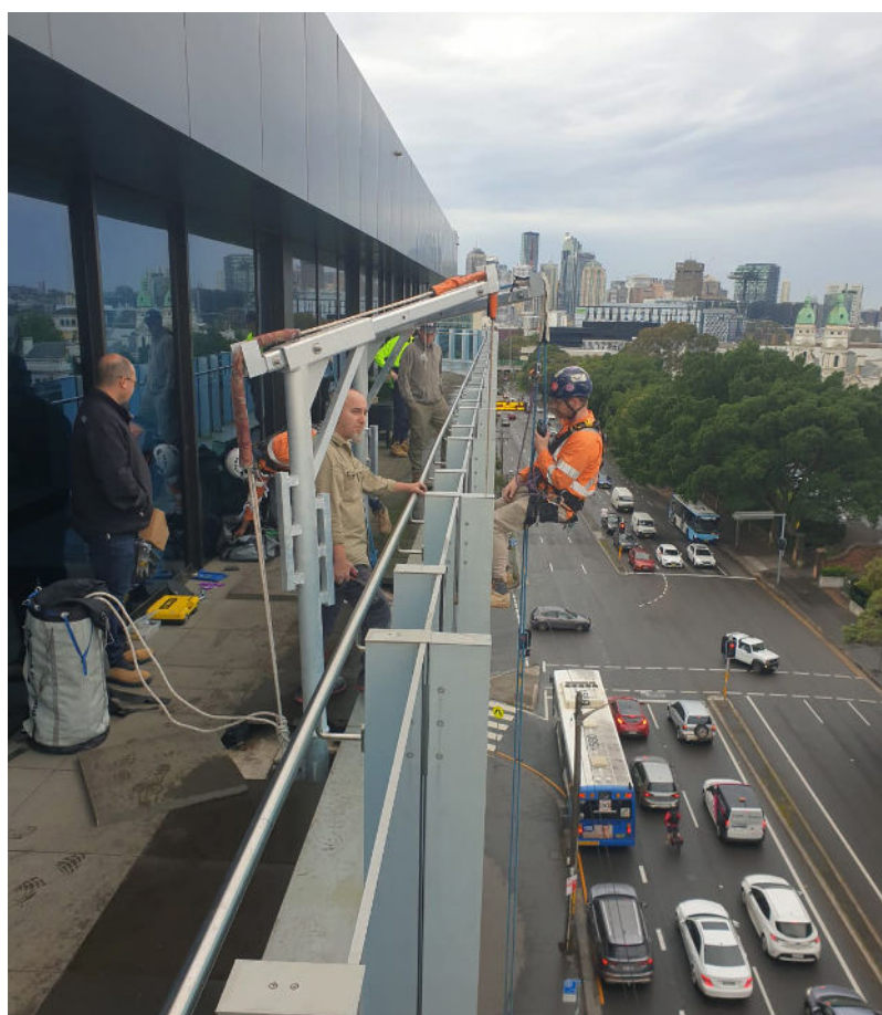
Using industrial rope access techniques
