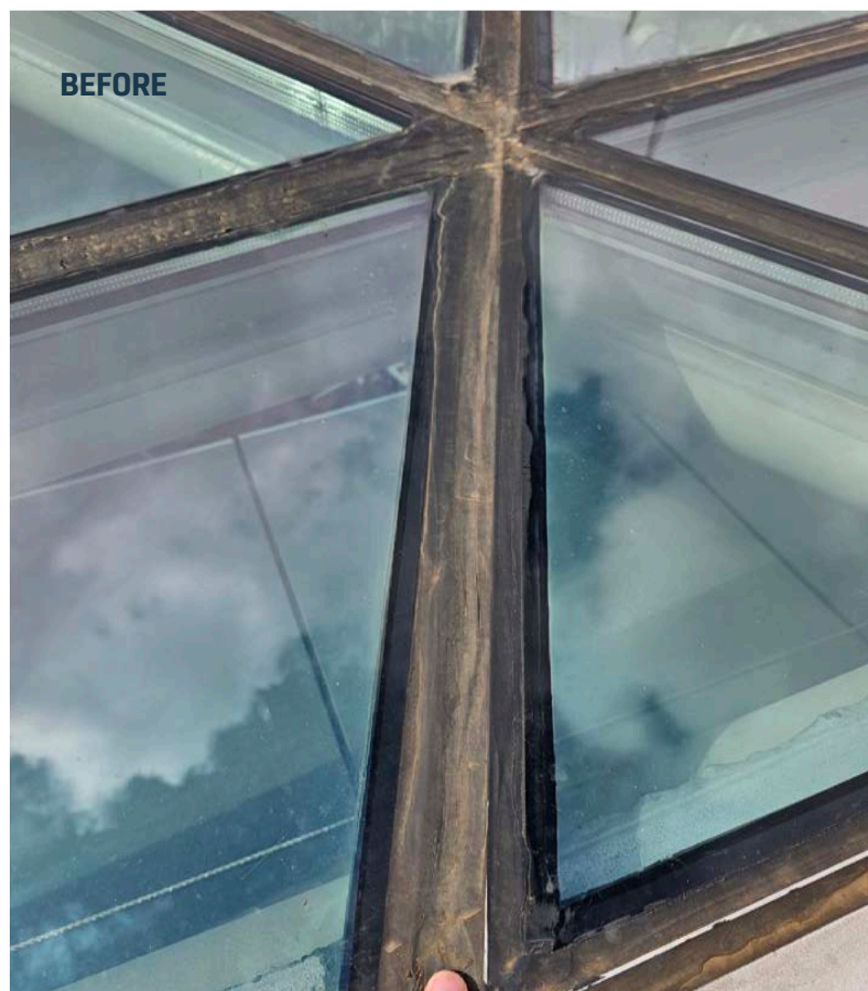
Before shot of the faded & leaking sealant
