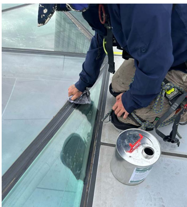
Applying the Tremco TREMGlaze 50.
