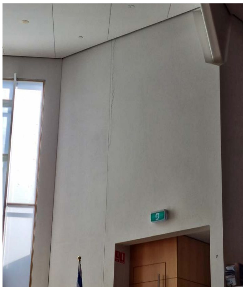
Water ingress damage on the inside of the atrium wall panels
