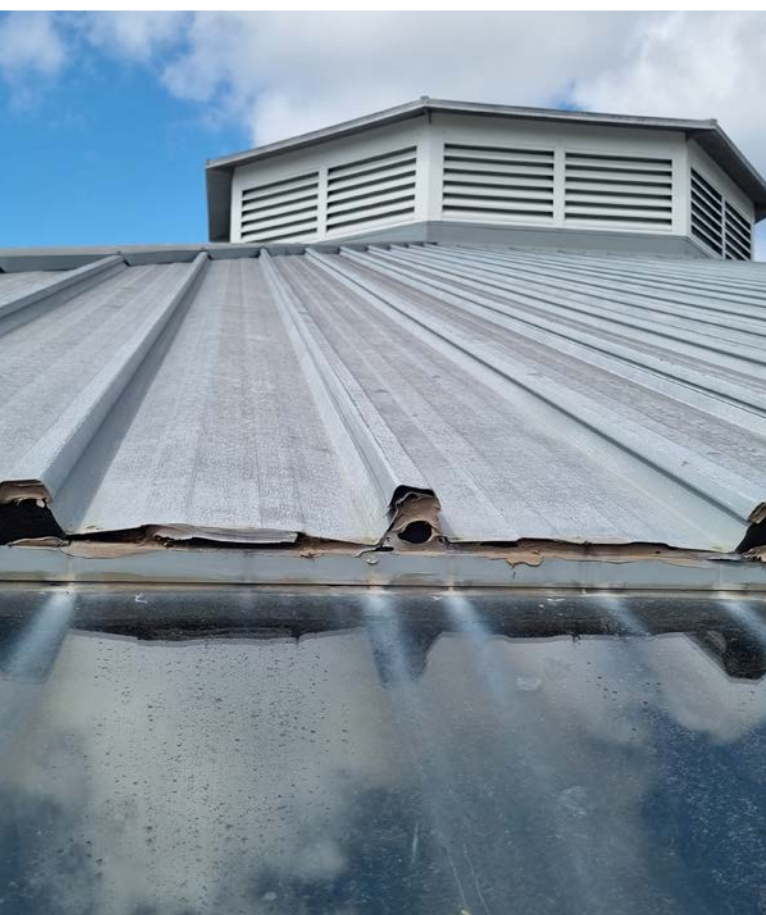
Inspection of perished barge capping to determine water ingress areas
