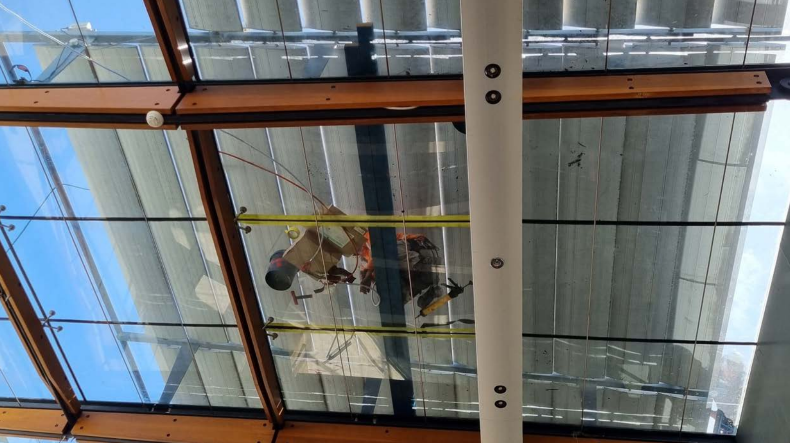
Our technicians in action applying the sealant
