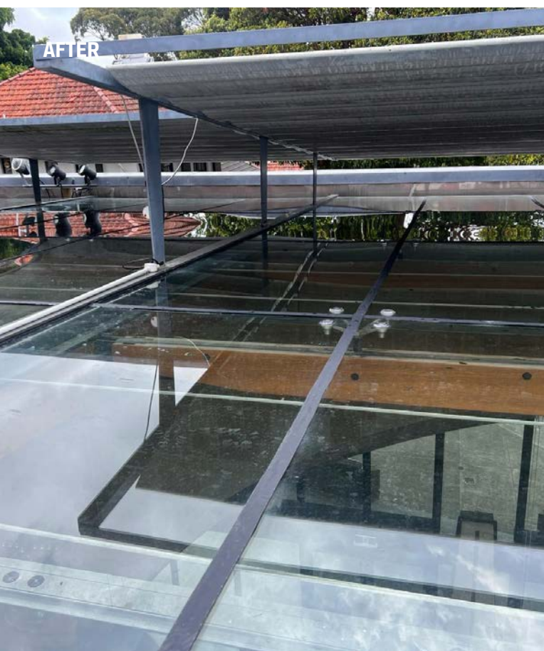
New sealant between all glass joints.
