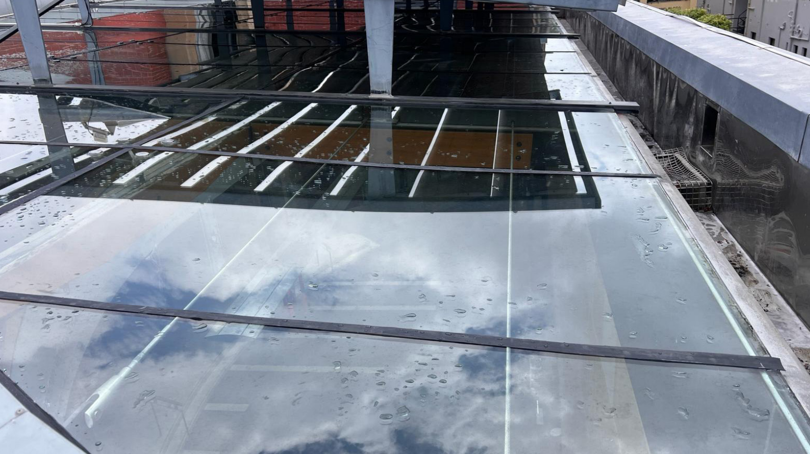
Effective application of the Tremco TREMGlaze 50 and Spectrem Simple Seal 1.5.
