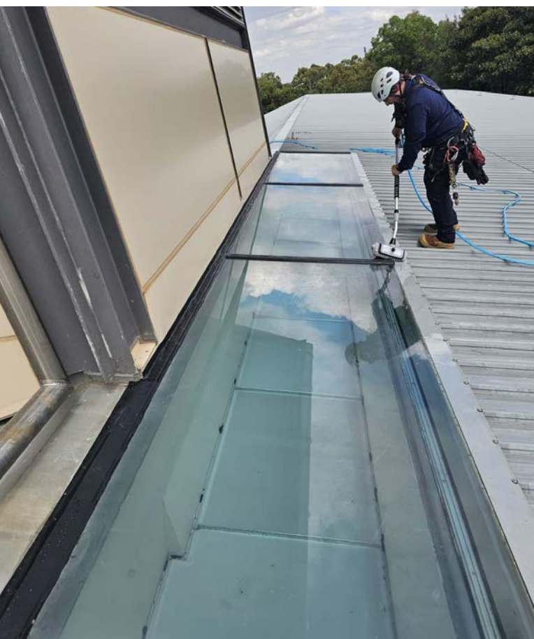
Surface preparation before applying Simple Seal
