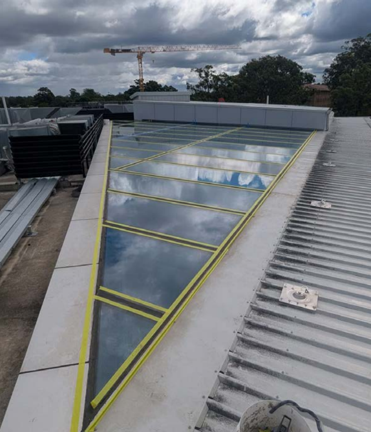
Surface preparation before applying Simple Seal
