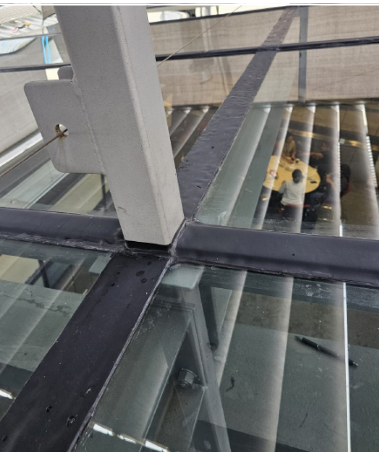
Applied Simple Seal to Atrium glass joints
