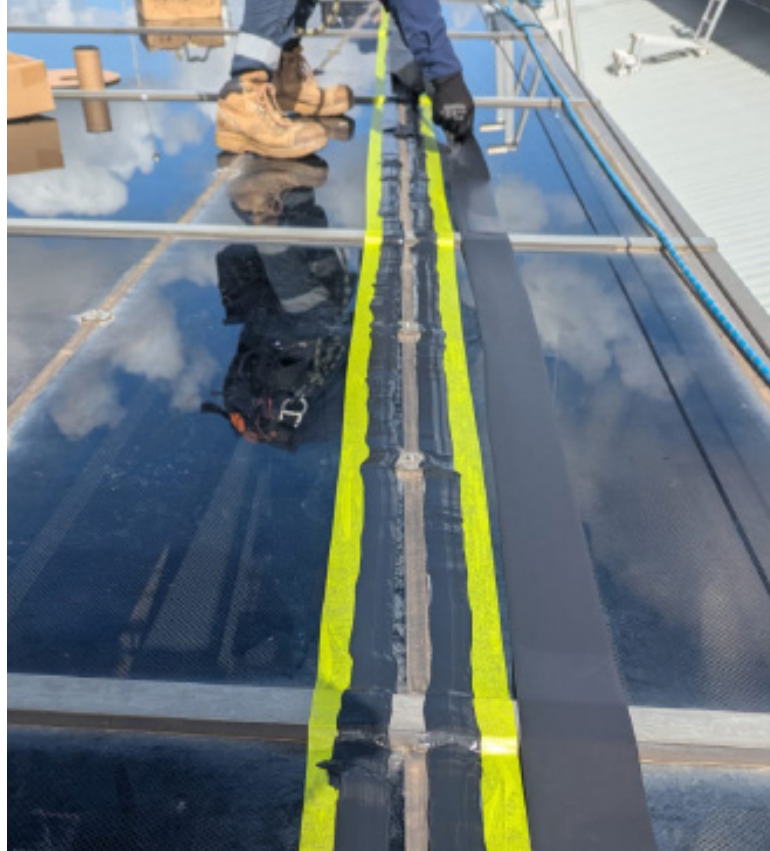
Applying the Tremco Simple Seal
