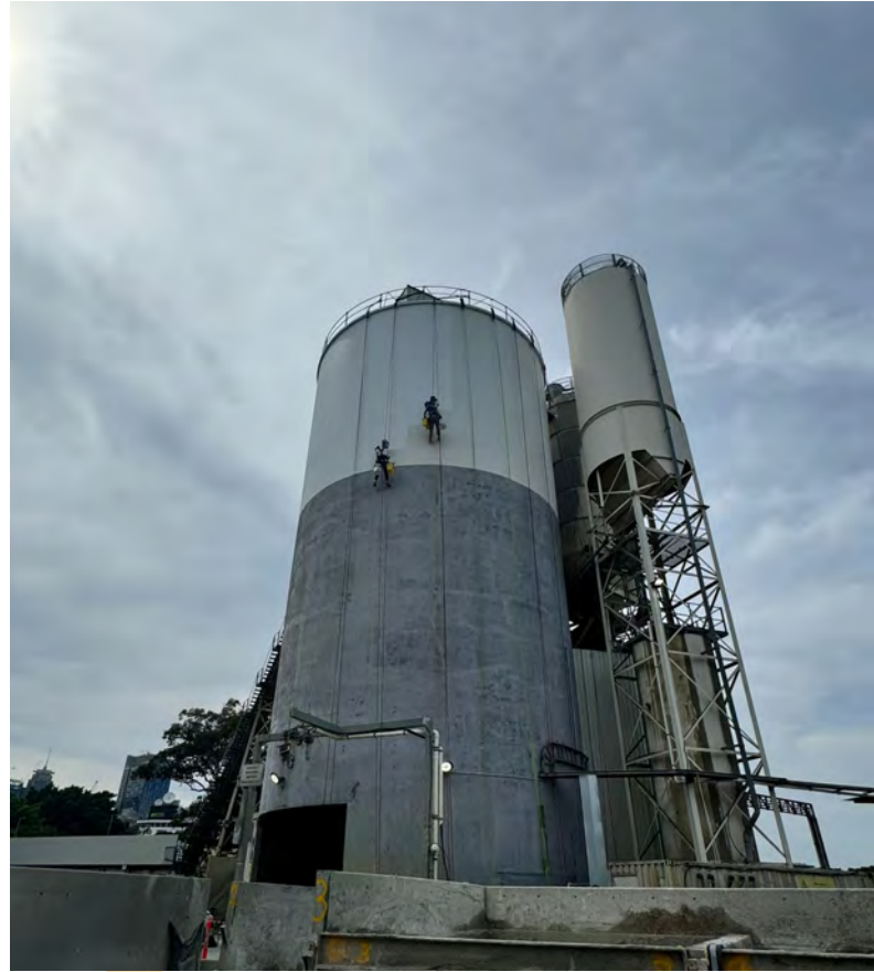
We installed additional rope access anchors points, allowing comprehensive and secure coverage across the entire silo structure
