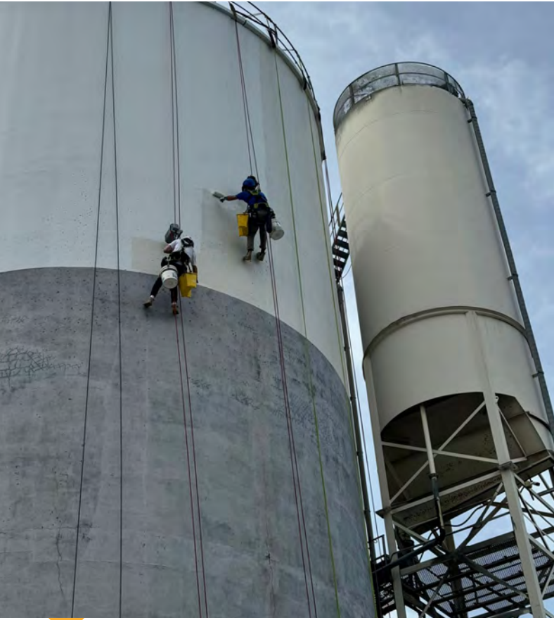
Applying Dulux protective coating systems
